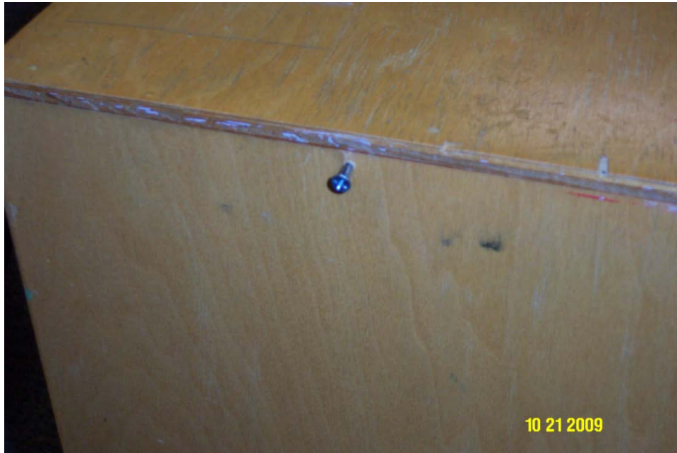
Photograph 1 – Taken in a classroom at the United Methodist facility on 10/21/2009 showing a screw protruding from a bookcase at child level.
