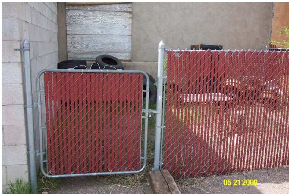
Photograph 4 – Taken at the Center facility on 5/21/2009 showing an enclosed area containing unsafe tires, rims, and a large metal cabinet. A child could access this area through the gap at the bottom of the gate.
