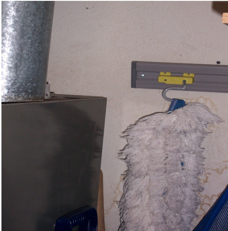
Photograph 1 – Taken at the Saguache facility on 5/20/2009 showing a cloth dust mop next to the furnace.
