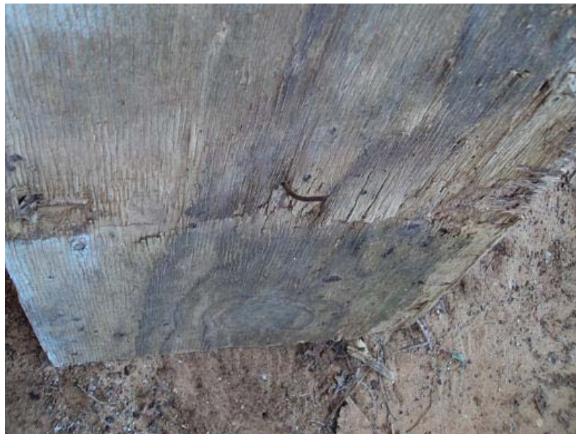
Photograph 4 – Taken at Foard County on 1/11/10 showing a nail protruding from a board on the playground.
