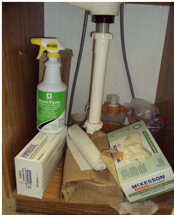
Photograph 12 – Taken at Turner on 1/12/10 showing cleaning solution with a label warning “KEEP OUT OF REACH OF CHILDREN” stored in an unlocked cabinet under a classroom sink.
