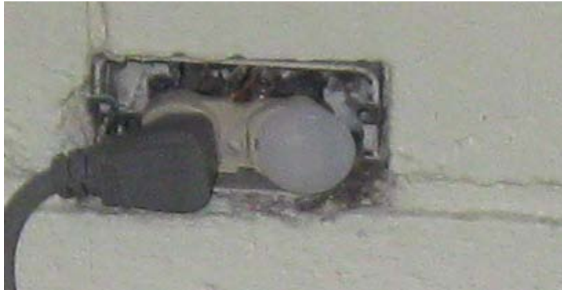
Photograph 2b – Taken at Comal No. 1 on 12/16/09 showing a closeup of the exposed outlet in Photograph 2a.
