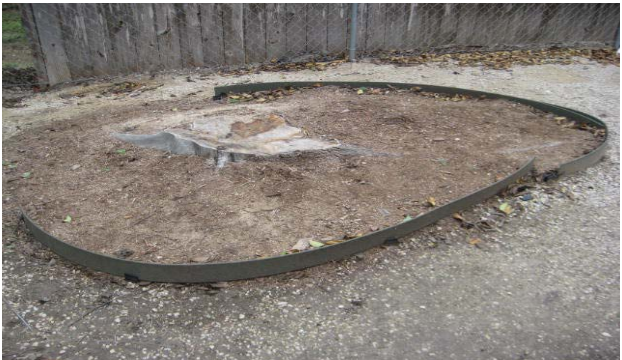
Photograph 7 – Taken at Comal No. 2 on 12/16/09 showing an exposed tree stump and surrounding plastic landscape edging in an area leading to the playground. The stump and edging were potential tripping hazards.
