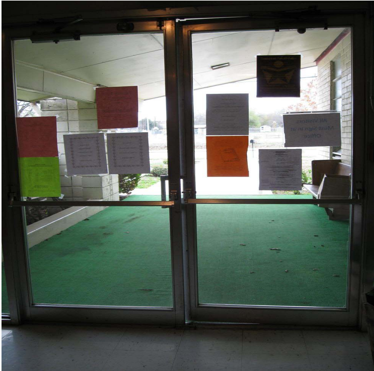
Photograph 4 – Taken at Comal No. 1 on 12/16/09 showing a side entrance with one of the double doors propped open. The doors, which opened to the street, allowed unrestricted access to the classrooms.
