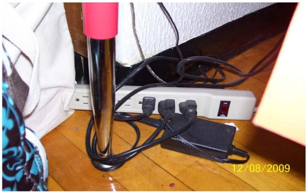
Photograph 7 – Taken at Fond du Lac on December 8, 2009, showing a power strip with exposed outlets on a classroom floor.
