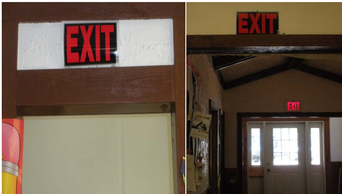
4/28/10 Corrected Photograph —exit signs posted
