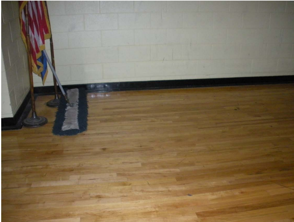
4/28/10 Corrected Photograph 3—Drywall and debris removed
