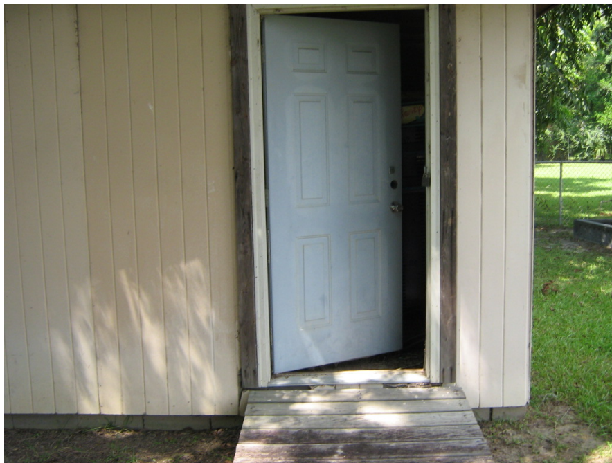
Photograph 4 – Taken at the Cook Head Start center on 8/25/2009 showing an unlocked shed on the playground. The shed was used to store potentially hazardous items, such as old equipment.
