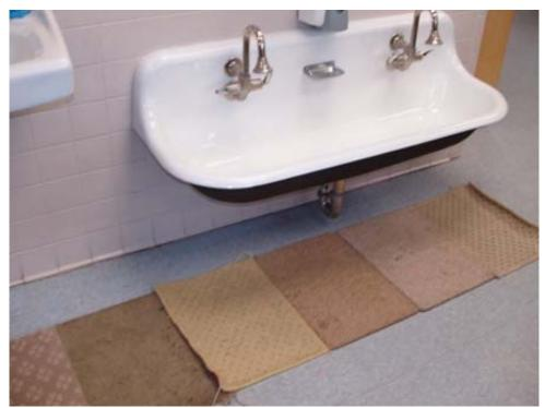
Photograph 3 – Taken at the Nathaniel Ely School on 6/3/09 showing six carpet squares that were pieced together and placed at the base of the children's sink in the classroom. The carpet presented a tripping hazard because it was curling up on the ends and not securely tacked to the floor.
