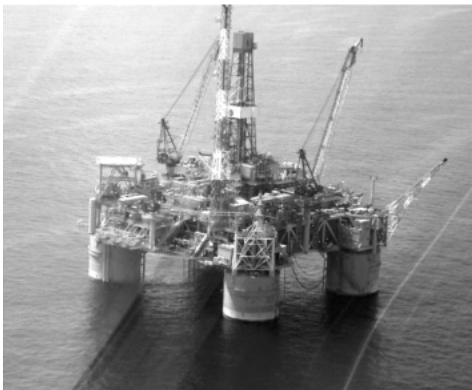
An off-shore platform in the Gulf of Mexico where NRC conducts unannounced inspections of well-logging activities.
