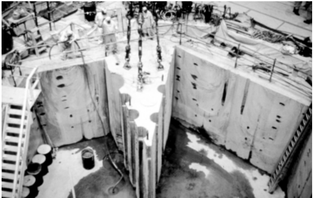
Decommissioning of the Ft. St. Vrain Reactor in Colorado
