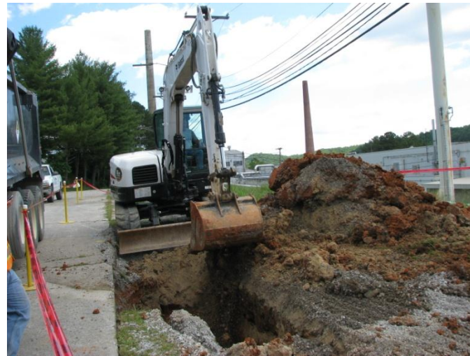
Excavating for PW Drain Pipe Removal
