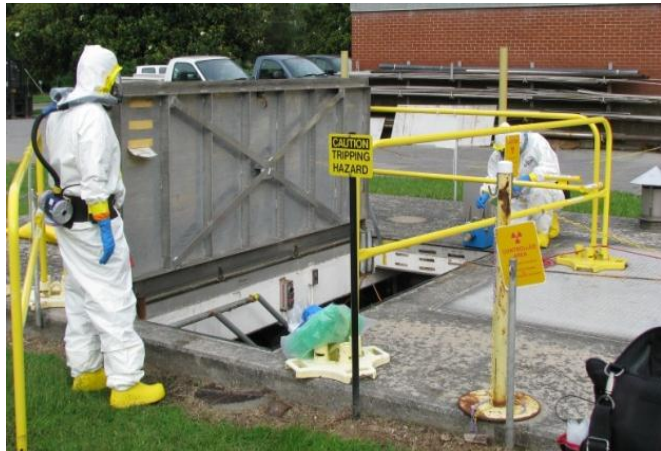
Preparing for 4556 Filter Pit Entry
