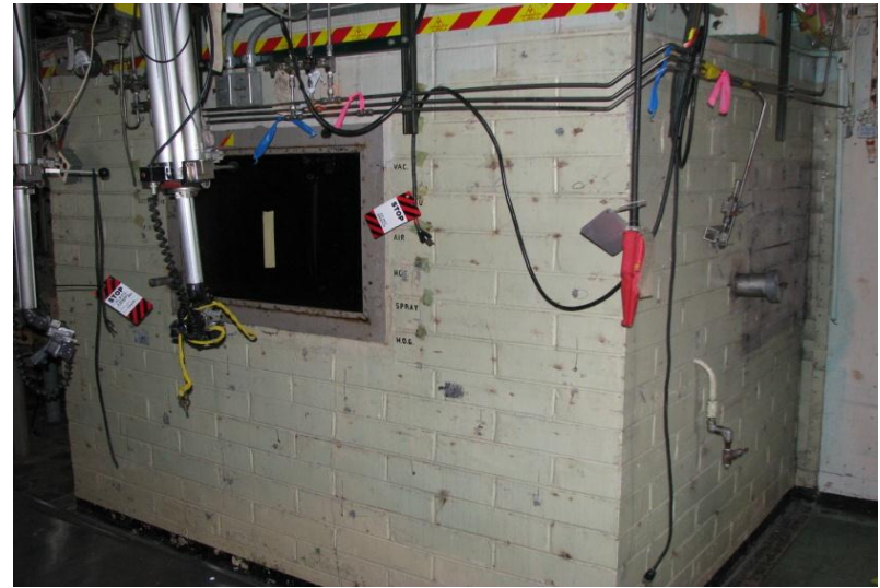
Building 3030 Hot Cell with Lead Shielding Removed
