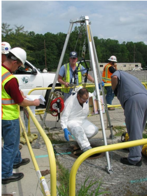
Making Confined Space Entry into Manhole Prior to Grouting
