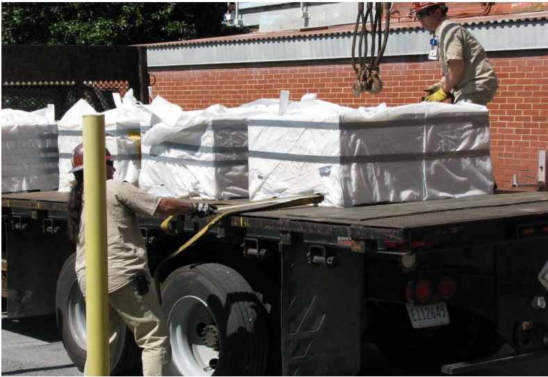
Preparing to Load Lead Shielding into Intermodal Container
