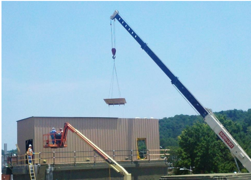
3026D Hot Cell Roof Access Enclosure Wind Barrier
