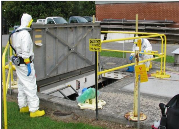
4556 Filter Pit Entry
