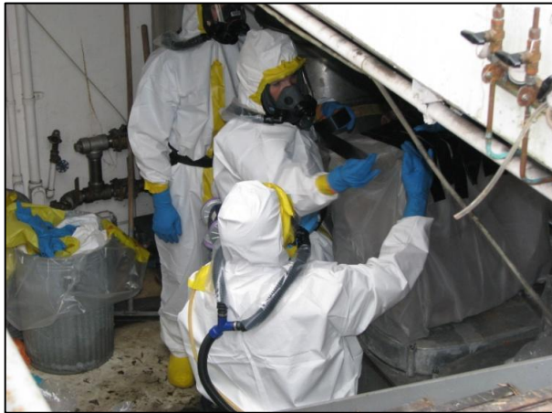
Removing HEPA Filter from 4556 Filter Pit Housing
