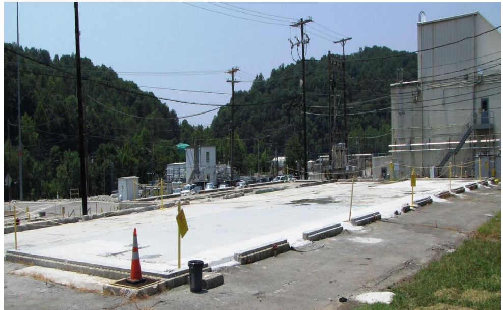
Former Building 3508 Slab
