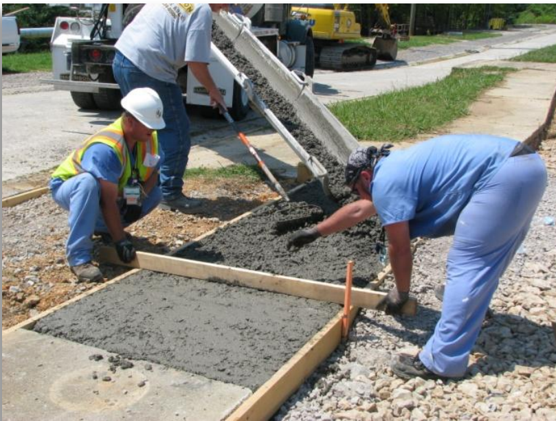
Sidewalk Repair at 2000
