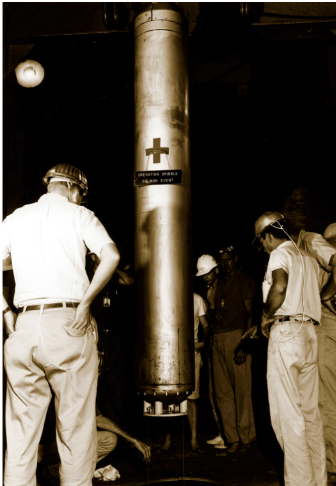
The 1964 Salmon Event, a 5-kiloton detonation conducted 280 meters deep in a Mississippi salt dome, confirmed the theory of decoupling as a means of concealing clandestine nuclear explosions. In this photo, experimenters are lowering a canister containing the nuclear explosive for the Salmon Event.
