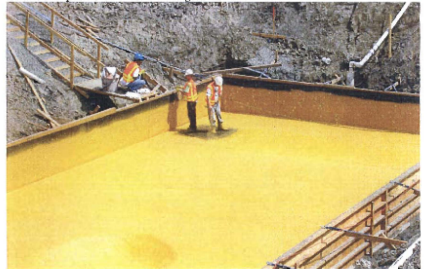
Below. Completion of 1 st coat of Integritank.
