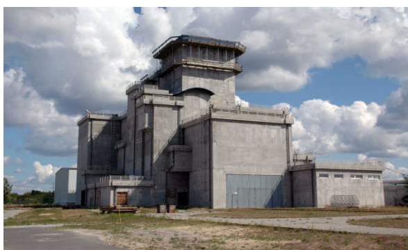
Figure 1: IFS-2 Spent Fuel Conditioning Facility.
