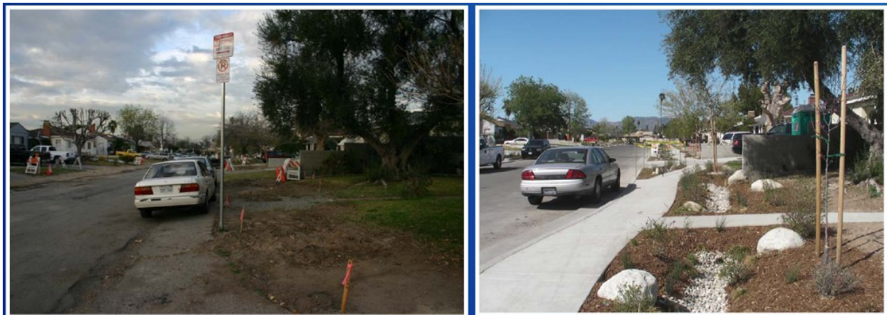
Elmer Avenue before and after Reclamation stormwater infrastructure upgrades. Photos by Council for Watershed Health
