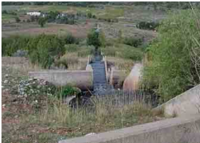
Drop Structure – Pine River Irrigation Project
