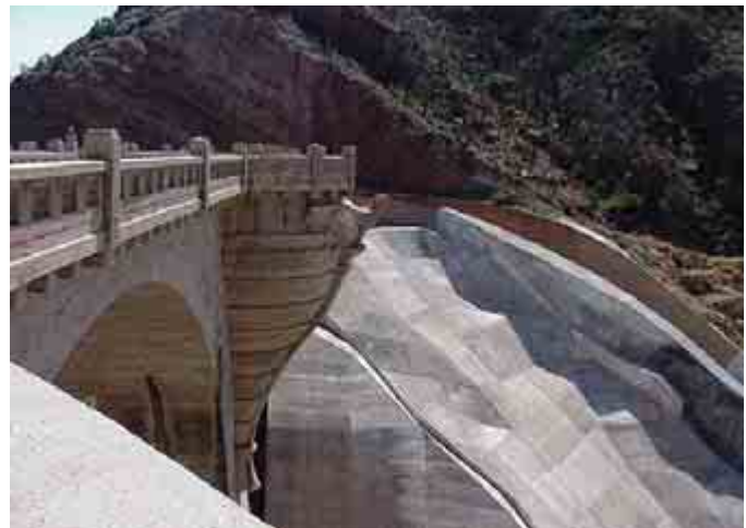
Coolidge Dam – San Carlos Irrigation Project
