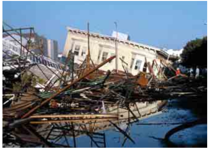
Loma Prieta earthquake, Beach and Divisadero Streets, Marina District, San Francisco, California, October 1989
