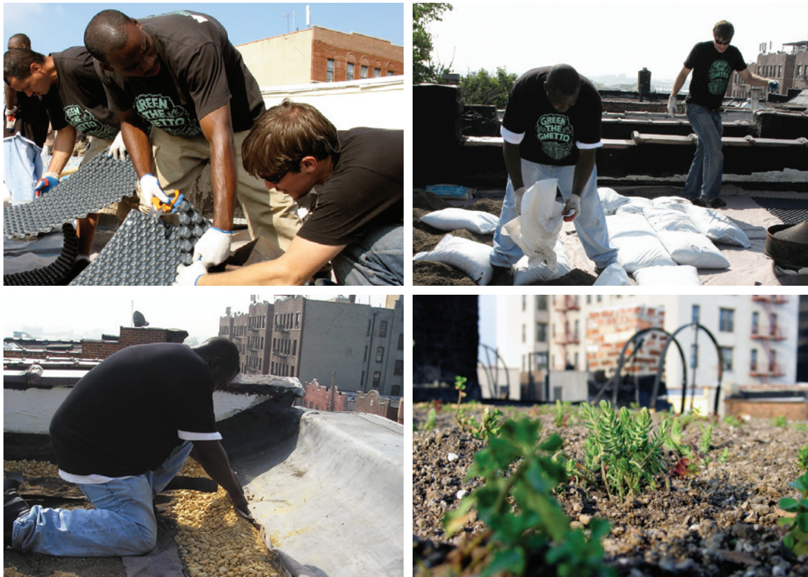
Figure 15: A Newly Installed Green Roof in New York City
