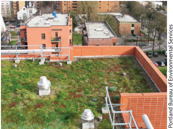
Figure 10: Green, or Eco, Roof in Portland, Oregon
