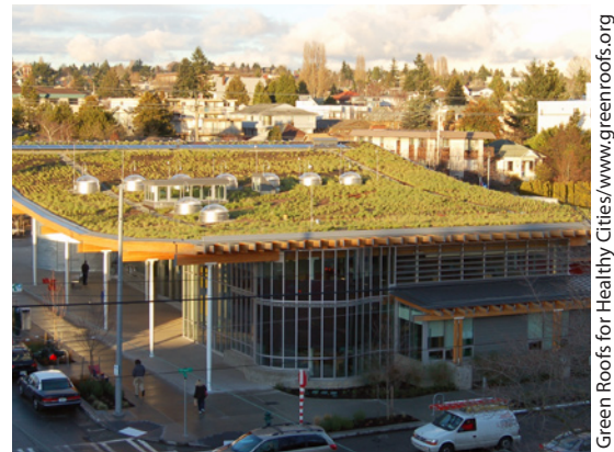
Figure 9: Green Roof on Seattle Public Library
