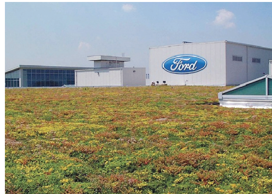
Figure 6: Ford’s Dearborn Truck Plant: An Example of an Extensive Green Roof
