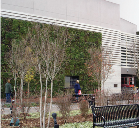
This 2,000-square foot (190 m 2 ) green wall on a store in Huntsville, Alabama, is one of the largest in North America. 14
