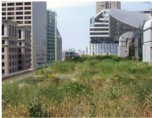
Figure 5: Combination Extensive/Intensive Green Roof—The Rooftop Garden on Chicago’s City Hall
