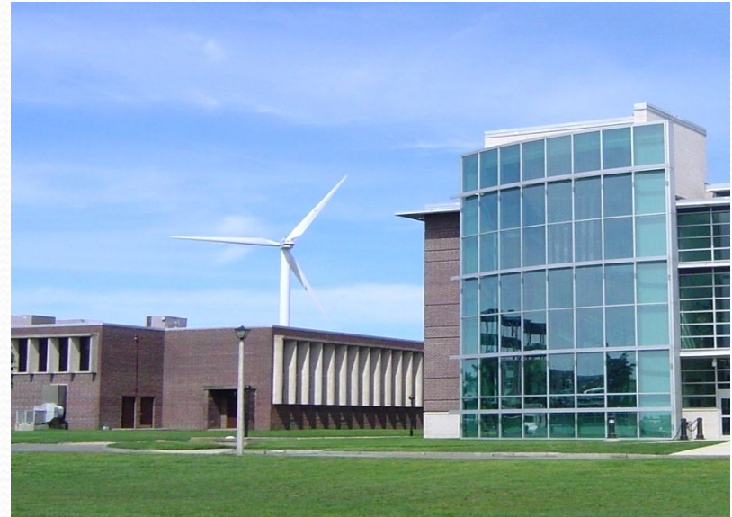
660 kW Wind Turbine @ Mass Maritime Academy
