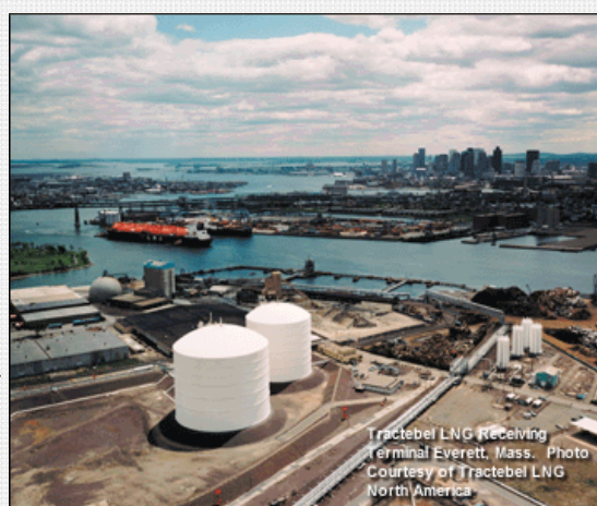
Figure IV-7 LNG Receiving Facility Everett, MA
