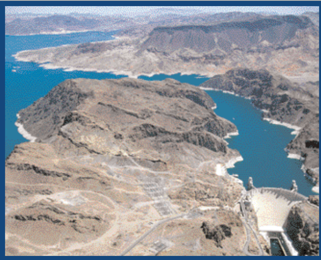
Aerial view of Hoover Dam and Lake Mead
