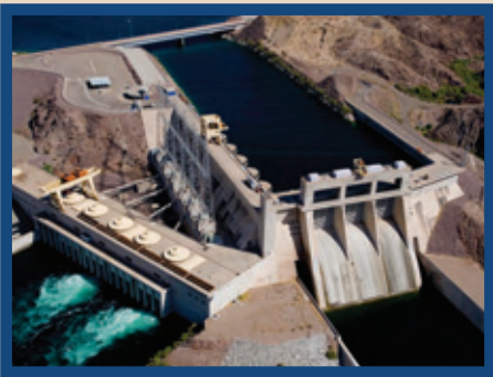
Davis Dam spillway
