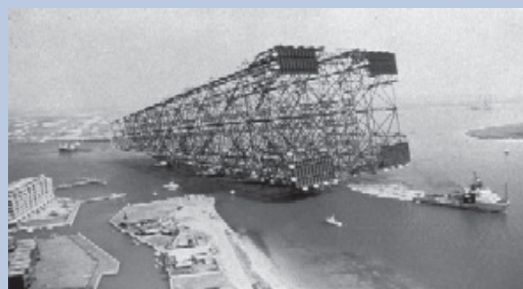
Figure 4. Shell's "Bullwinkle" Platform; World's Tallest Pile Supported Steel Platform (1,736 feet in total height)
