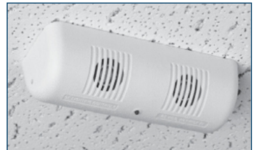
Ceiling occupancy sensor
