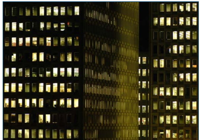
Automatic whole building lighting controls can reduce after hours lighting waste!
