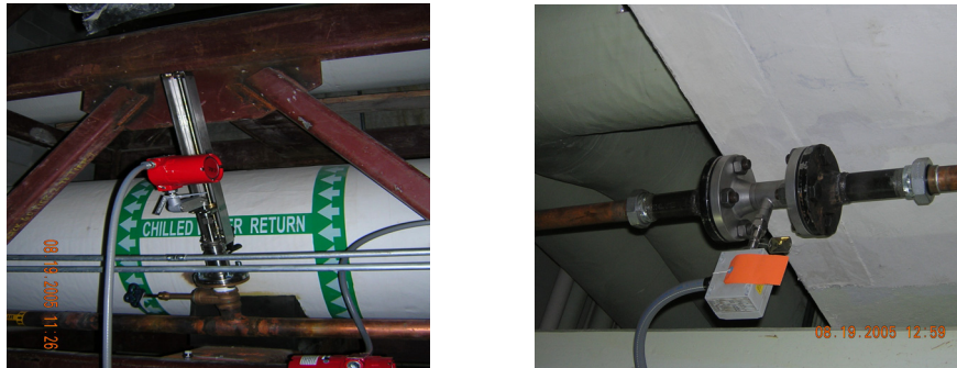
Figure 8.7. Compressed Air Meter Applications at the NIH. Meter in left photo is an insertion-type while meter in right photo is an in-line-type.
