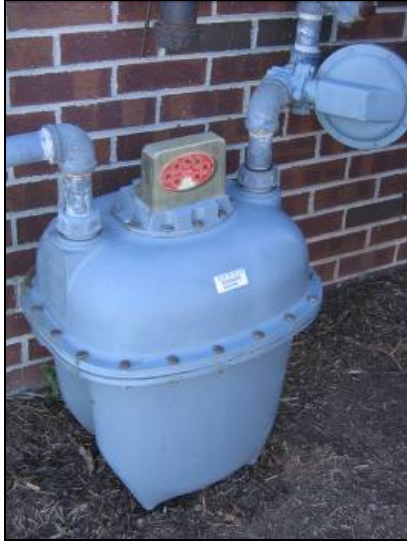
Figure 5.1. Typical Natural Gas Diaphragm Meter
