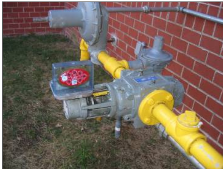
Figure 5.2. Typical Natural Gas Rotary Flow Meter
