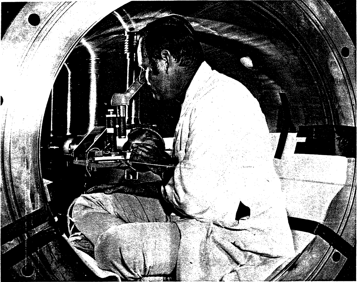
FIGURE III.2.g.5 Final drift-tube adjustment (interior).
