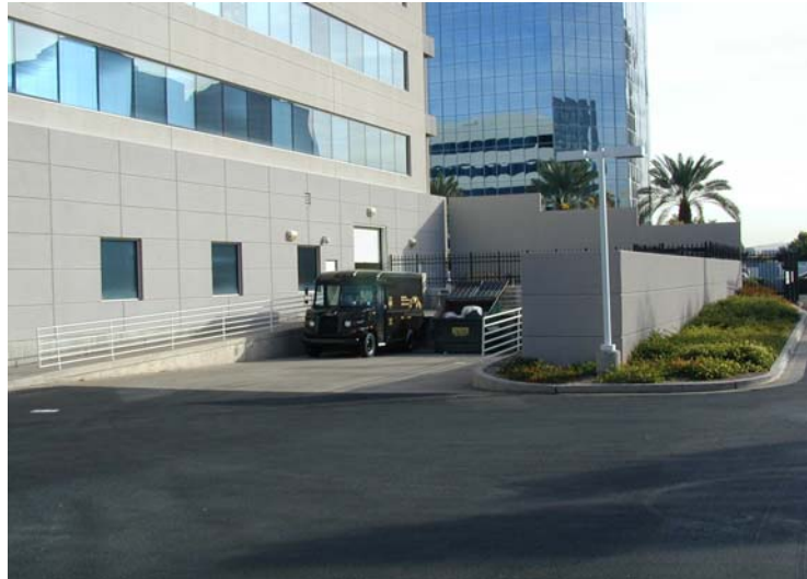
Figure 4: Unguarded loading dock at shared driveway.
