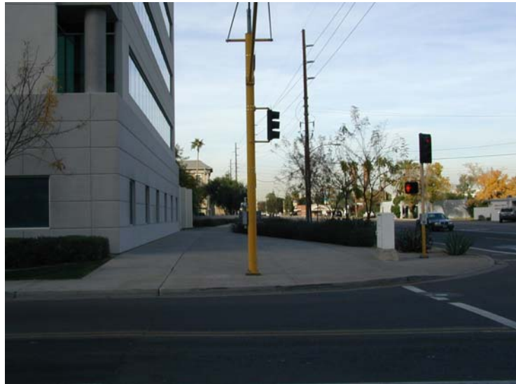
Figure 2: Stationary bollards not in place.
