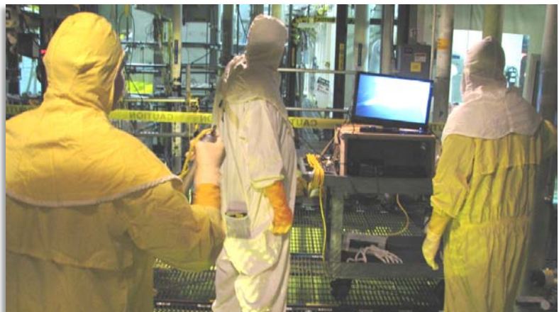
Knockout Pot Pretreatment Operations at 100K
