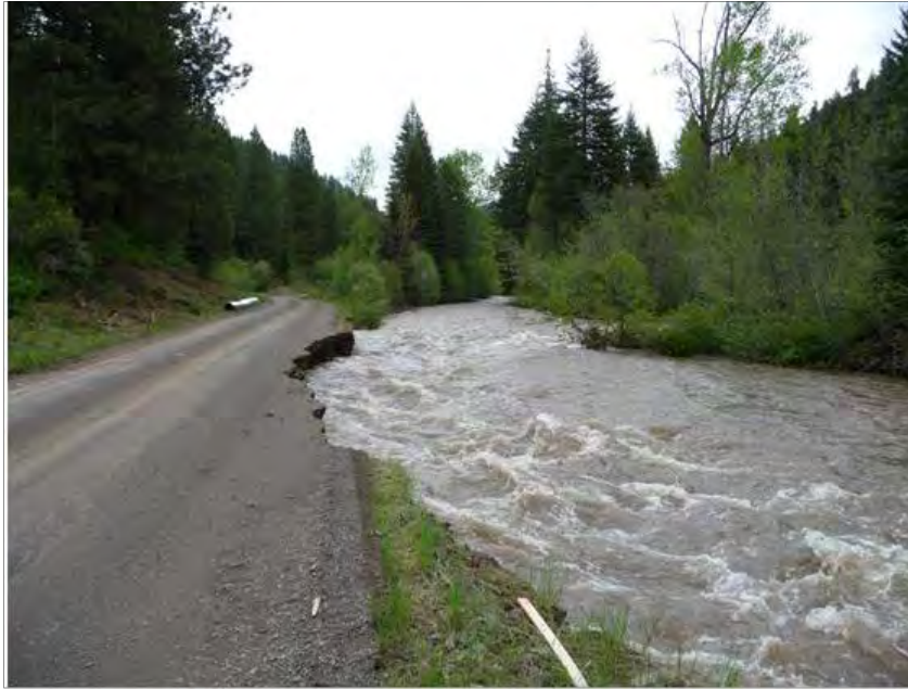
BEFORE: Oregon (FS Photo). A section of FS Road 7785 had washed out due to flooding.
