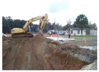
Two USTs were removed to eliminate releases into the soil and groundwater. Due to the extensive amount of clay at this site, it was necessary to remove additional soil before a no further action approval was received from regulators. This site at Wright Army Airfield is now part of a 'Joint-use Airfield' benefiting the Army and Liberty County.
