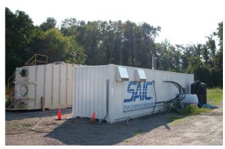
A pilot-scale product recovery system consisting of a combination of a surfactant called Petrosolv<sup>TM</sup> and a multiphase extraction system was implemented to recover freephase product from under a 500,000 gallon aboveground storage tank (AST).
