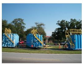
A pilot-study tracer system was implemented to determine the feasibility of the proposed corrective action by the remediation contractor. An eosine, fluorescein, and rhodamine solution was injected into the deeper zone of a Trichloroethylene plume to trace the dispersion radius.
