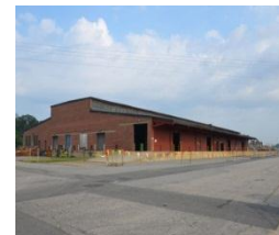
Figure 1: Warehouse undergoing demolition.
