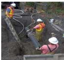
Figure 5: Workers replace water distribution system
