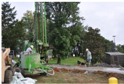
Figure 3: Workers install wells utilized by energy efficient ground source heat pumps.
