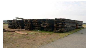
Figure 2: Demolished warehouse wooden beams segregated for recycling.
