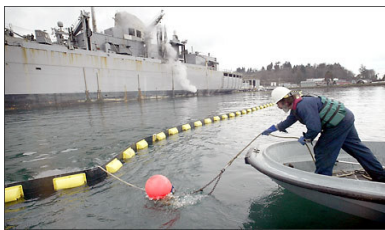
Setting boom prior to fueling USS Sacramento at Manchester Fuel Depot
