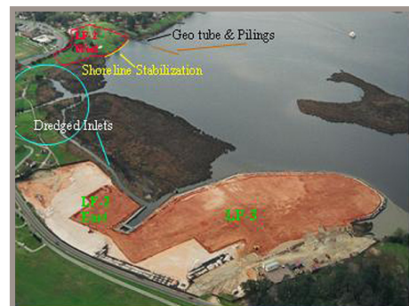
Aerial view showing proximities of LF 2 and LF 3
