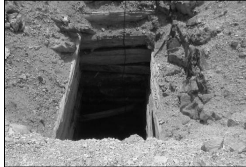
Water filled open shaft located along a high use 4 wheel drive road in San Juan County, Colorado.
