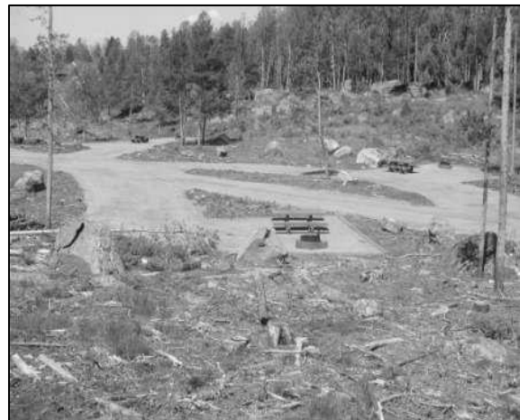
Scab Creek Campground after ARRA Construction
