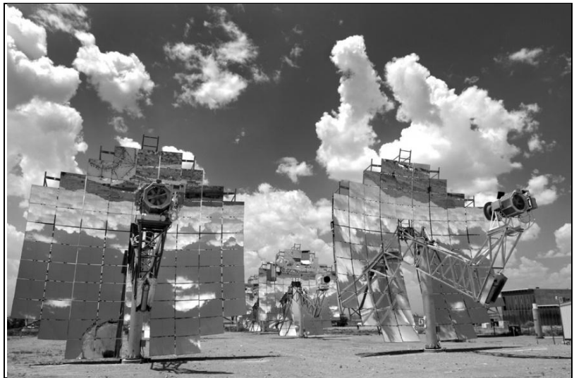
As of December 2010, the first quarter of fiscal year 2011, the Bureau of Land Management had approved nine large-scale solar energy projects – the first to be built on U.S. public lands in California and Nevada – that, cumulatively, will generate more than 3,600 megawatts of electricity. Two of these projects will use 38-foot wide dishes with solar receivers and engines, similar to those shown above.
