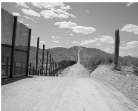
Southwest Border Fence
