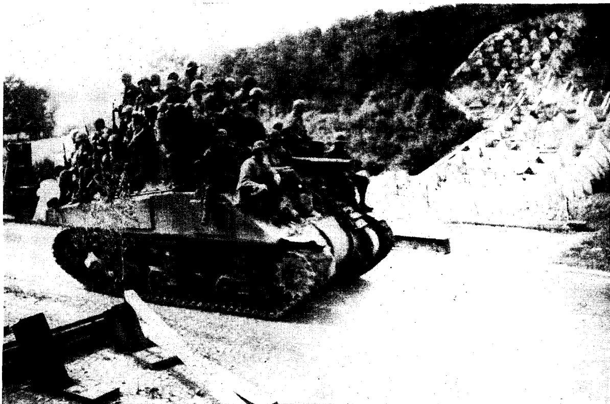
Figure 21.—Line of dragon's teeth of Westwall. Note steel antitank barrier set at an angle in the road.
