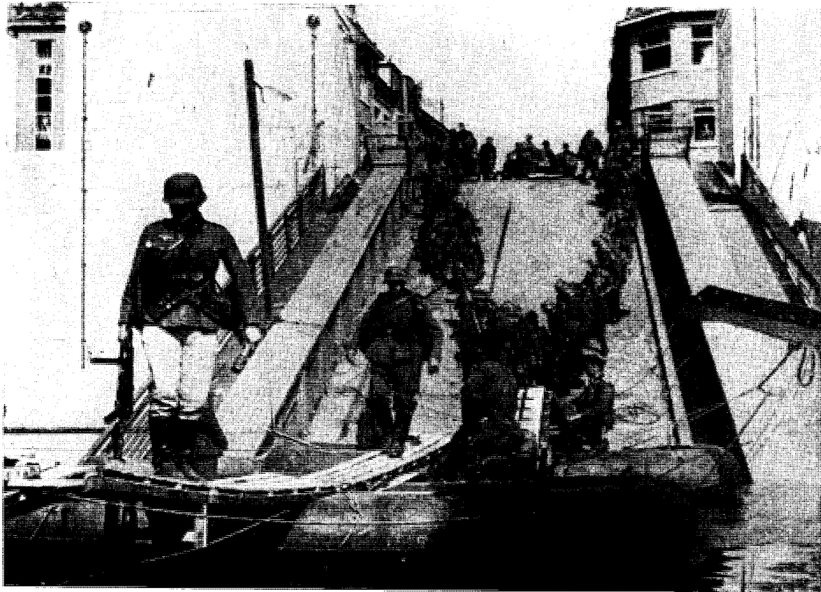
Figure 96.—Track bridge and medium pneumatic boat.
