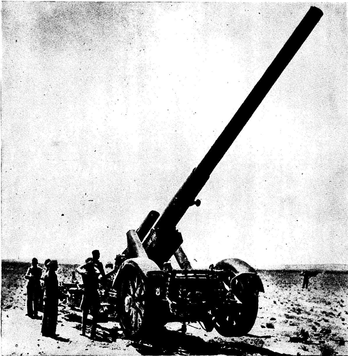
Figure 42.—17 cm K. in Mrs. Laf. (170-mm gun mounted on 210-mm howitzer carriage).
