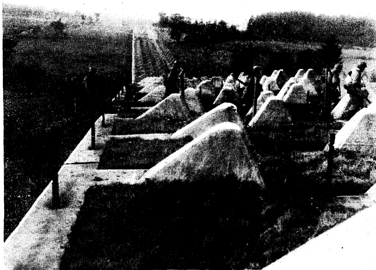
Figure 16.--Dragon's teeth showing concrete foundations.
