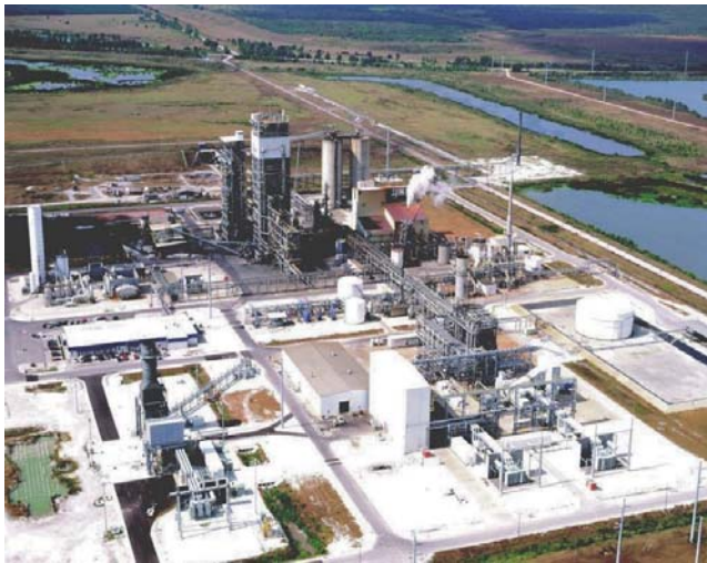
Polk Power Station: IGCC Plant in Tampa, FL (250 MW)
