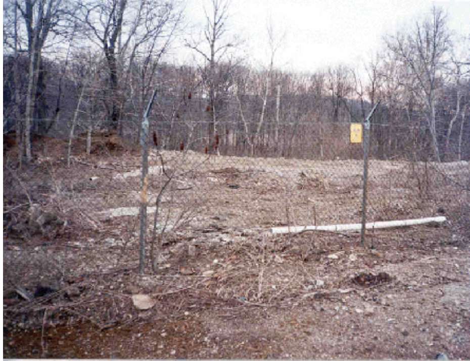
Figure 1-5. Top of slag pile at Site C . The slag is found below the cleared area and it is covered with approximately 0.5 m to 1 m (1.5 ft to 3 ft) of soil and construction debris.
