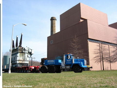
Figure 4-15. Top photo is transformer with EHV bushings and external oil cooling radiators removed for transport. Bottom photo is 230kV class transformer being relocated at a power plant site. The smaller size of this transformer and the short distance of move (within the power plant property) did not require removing HV Bushings from transformer.
