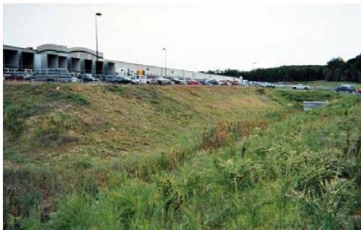
A bioretention stormwater management system designed to treat rooftop and parking lot runoff, Cecil County, Maryland (EPA OIG Photo)
