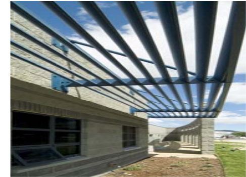
Reno ANGB (shading in building design)
