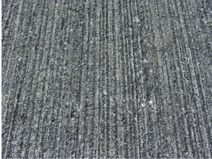
Figure 4. Concrete Surface of Figure-Eight Course
