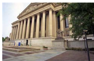
National Archives Building, Washington, DC
