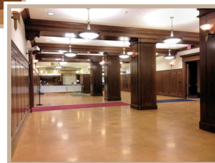
New cork floor in what will be the Research Commons area
