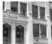
FIGURE 10 Exterior view of blast windows fabricated with custom muntin placing upper and lower panes in separate planes to simulate the appearance of double hung windows. (Mariah McGaughey/GSA)
