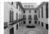
FIGURE 12 Thoughtful analysis to balance GSA preservation, cost, and performance goals supported historic window retention with replacement of non-historic windows at this 1930 courthouse. Blast-resistant, thermal storm windows were installed where original windows remained on courtrooms and the upper and lower levels of the light court. Roman arched windows in the light court were determined to meet blast protection requirements and did not require storm windows. Non-historic windows on the exterior facades were replaced with new blast resistant windows carefully replicating the building's original windows. (Carol M. Highsmith Photography, Inc./GSA)
