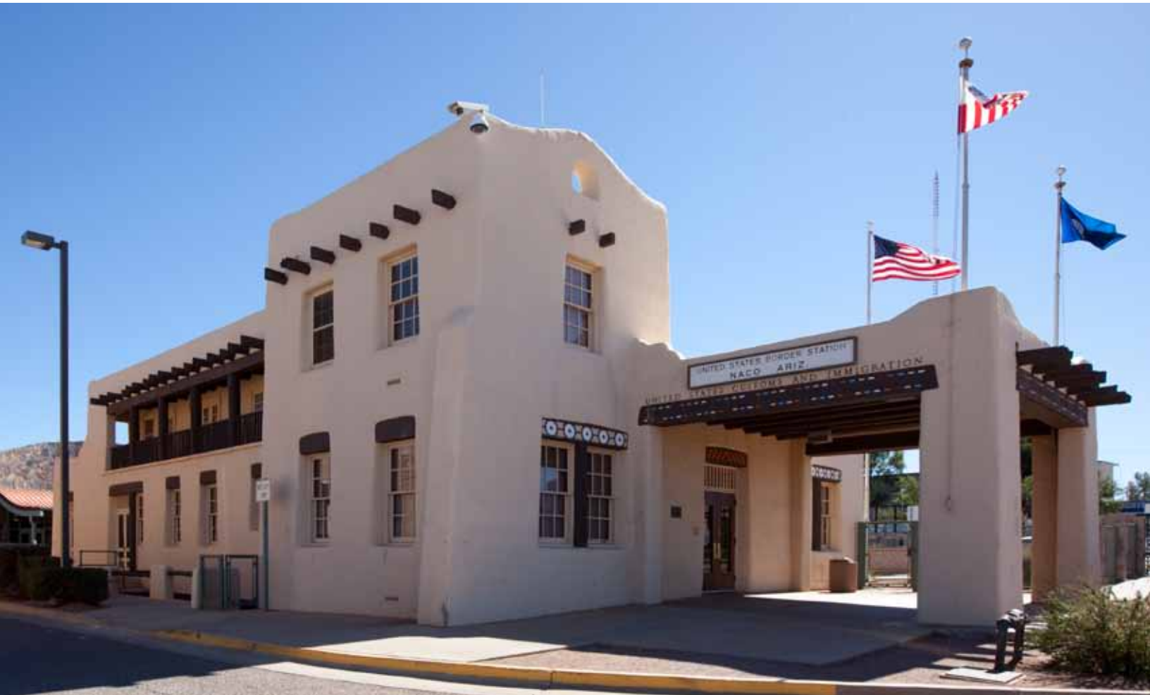
U.S. BORDER INSPECTION STATION NACO, ARIZONA
