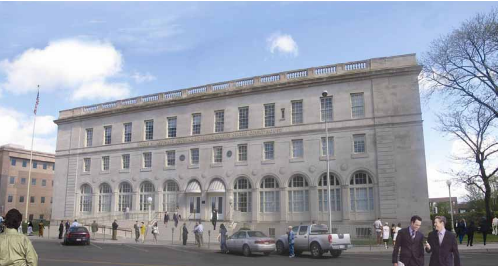
WAYNE N. ASPINALL FEDERAL BUILDING AND U.S. COURTHOUSE GRAND JUNCTION, COLORADO
