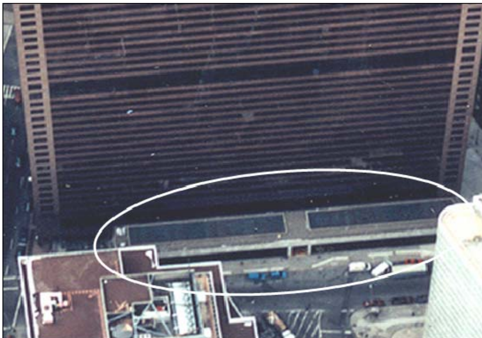
Figure 1–4. Aerial view from the north side of WTC 7, showing the Con Edison substation.
