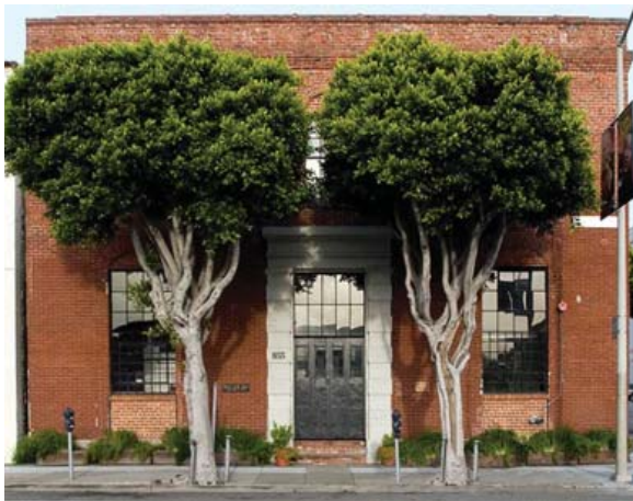
One of a number of historic commercial properties in a historic district renovated by the Ron Kaufman Co., the 1855 Gibb-Sanborn Warehouse, a rare city survivor of the Gold Rush era, is protected by an easement held by San Francisco Architectural Heritage. Photo: ©SF Architectural Heritage.
