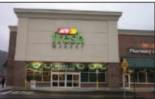
Photo Courtesy of Solar Turbines
