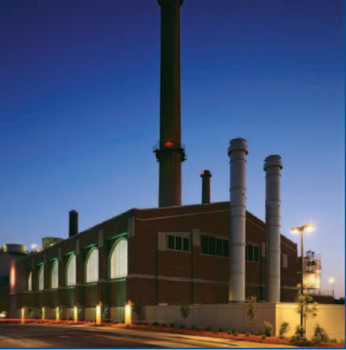
CHP District Energy System, University of Missouri at Columbia, Courtesy of IDEA
