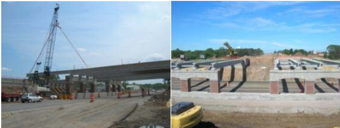
Figure 6. McKnight Road bridges under construction.
