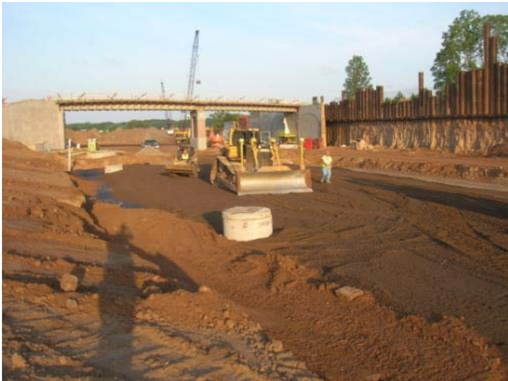
Figure 8. Pedestrian bridge under construction.
