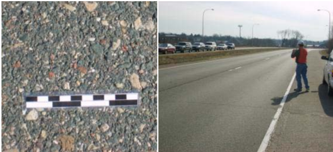
Figure 12. Existing TH 36 HMA pavement.
