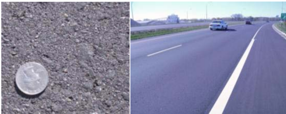
Figure 13. Newly constructed TH 36 HMA pavement.
