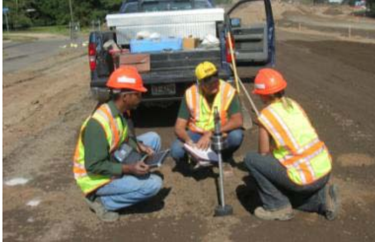
Figure 11. Technicians check the embankment compaction with an LWD. (Source: Mn/DOT)
