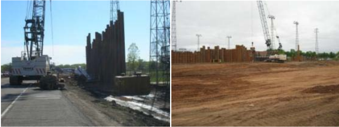
Figure 5. Shoring being placed along TH 36.
