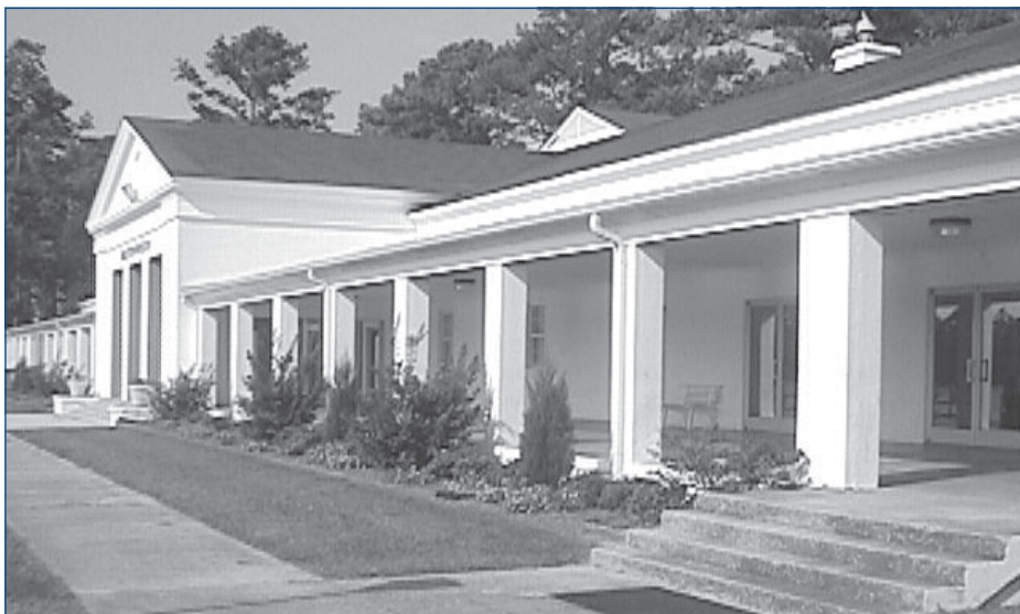
GHPs were determined to be the most cost-effective option available to replace the old, ineffective HVAC system in Marston Pavilion, a historic building and community center for a U.S. Marine Corps base. The new GHP system costs 60 percent less to operate than the old system and provides excellent air quality and thermal comfort for the building.
