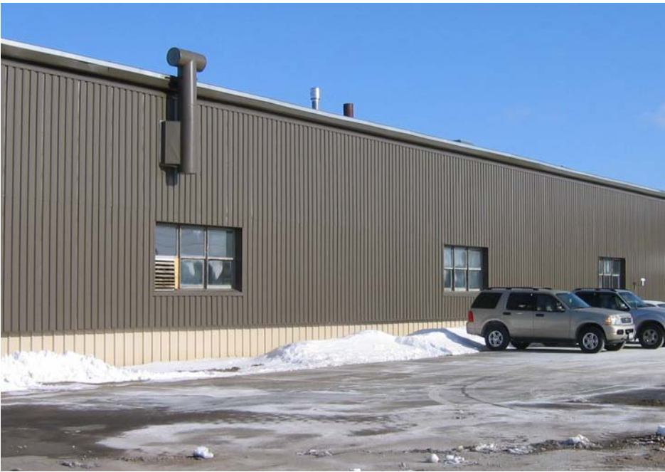
Transpired collector mounted on the south wall of the building. Photo by Ed Hancock, NREL/PIX 19363
