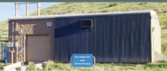
The transpired solar collector on the National Renewable Energy Laboratory's Waste Handling Facility in Golden, Colorado. Photo by Sheila Hayter, NREL/PIX 14003
